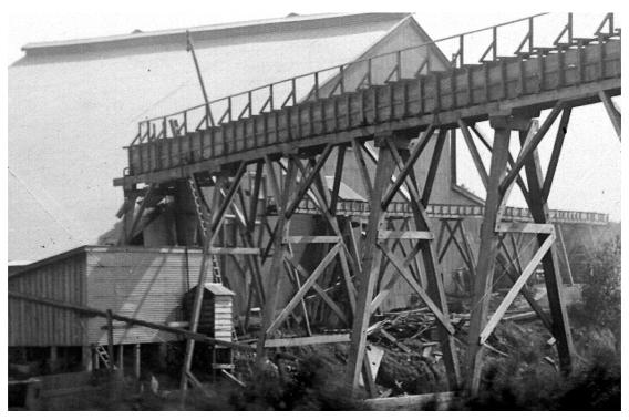
Detail. The large turbine pipe can just be made out near the left hand end of the large wooden flume. The much smaller flume in background may have been the terminus of a Mangatoetoe water race.
