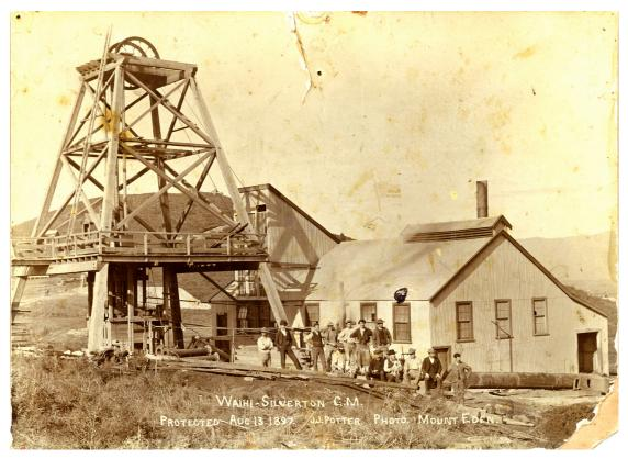
Silverton Shaft 1897. The building housed a wood fired boiler, winding engine, and pumping engine. There are 13 men and two dogs pictured here. Behind the men are squared mine props ready to be taken below. Behind the poppet legs is a mullock tip from the Gladstone shaft, and at the very right of the photograph can be seen (just) the Union No. 2 Shaft poppet. WACMA.
