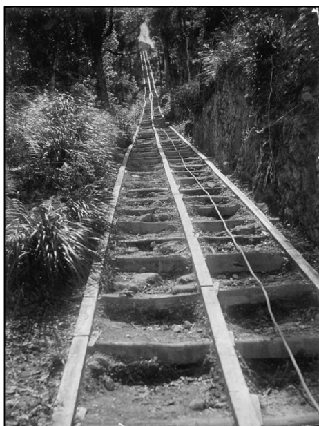
This is the Earl of Glasgow incline, but the County incline would have looked similar.
